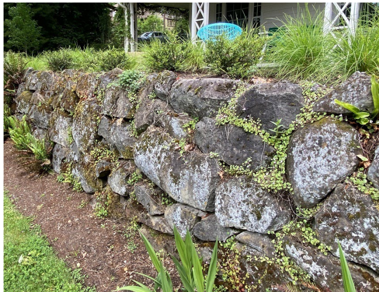
Terraced walls break up the continuity of fuels
