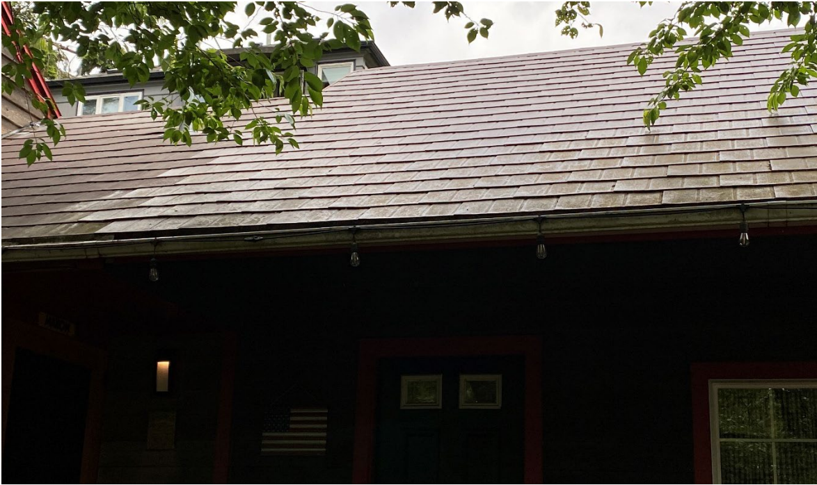
Metal roofing and gutters
